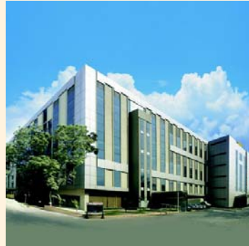
Switchgear Factory, Mumbai
