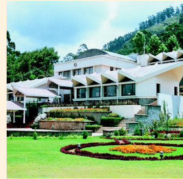
Switchgear Training Center, Coonoor
