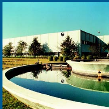
Switchgear Factory, Ahmednagar
