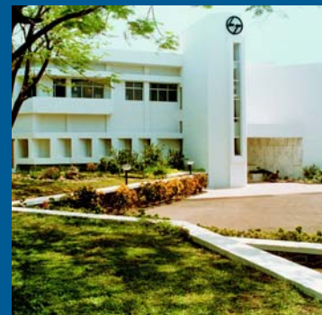
Switchgear Training Center, Pune
