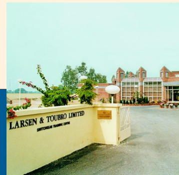
Switchgear Training Center, Lucknow
